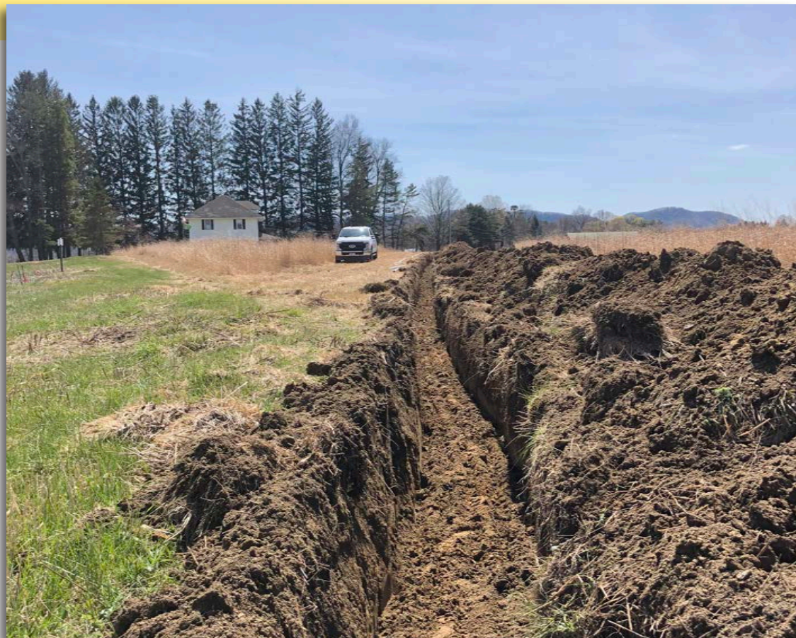
Staff and a contractor dug this trench to run the conduit
