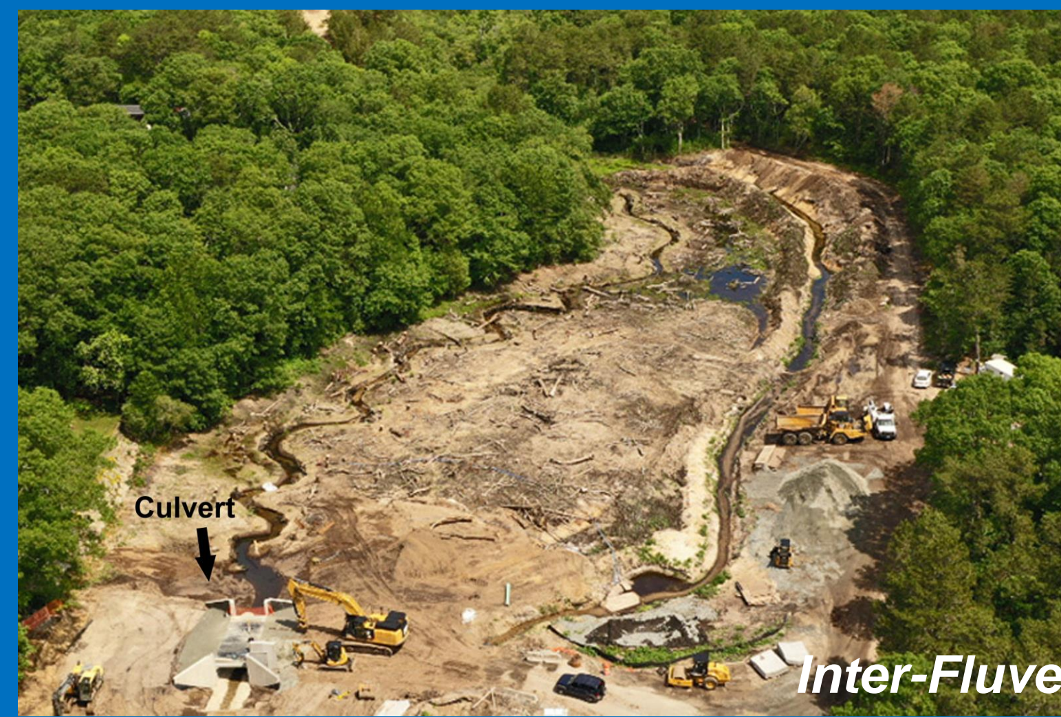
June 2021 – Culvert in Place
