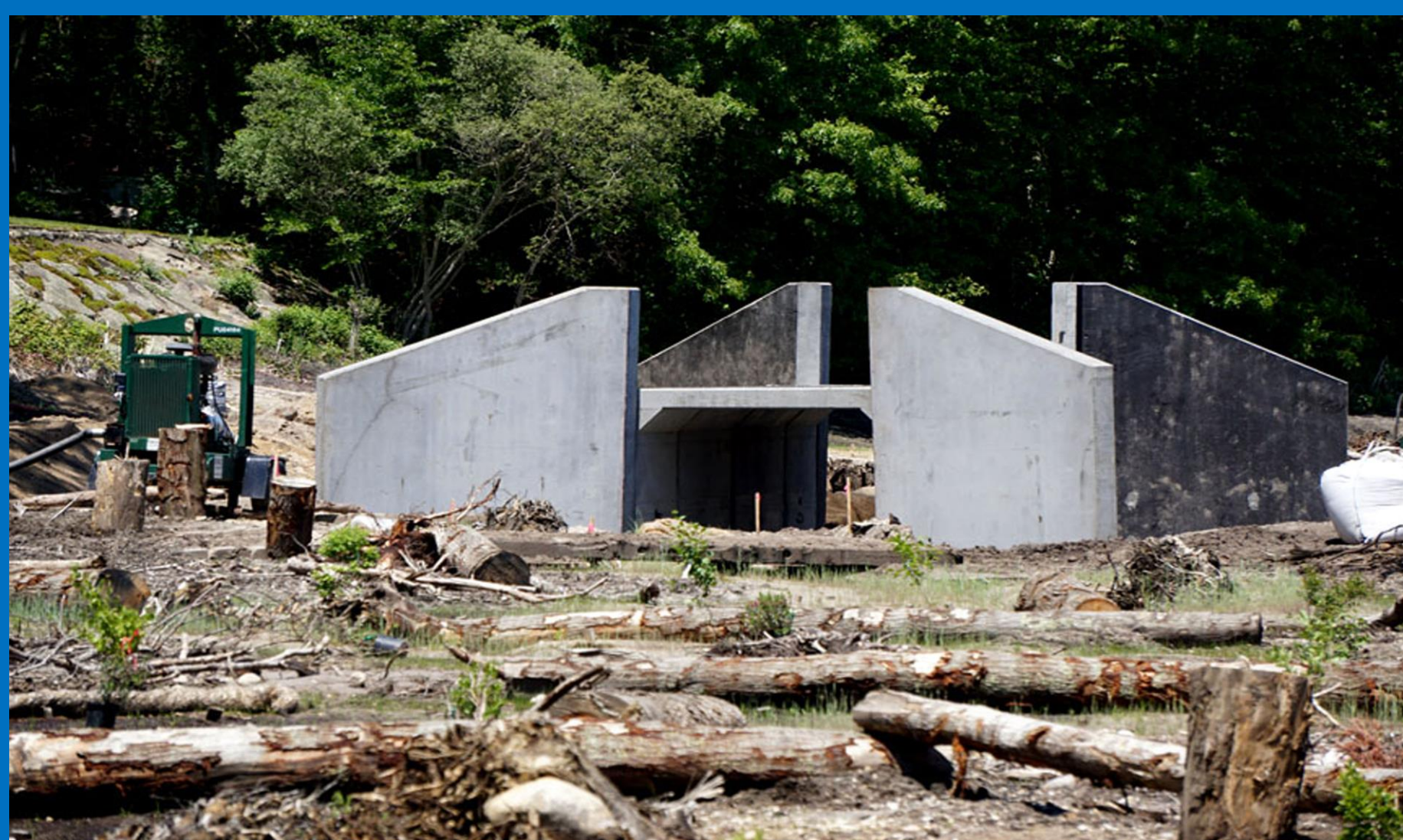
June 2021 – New Culvert in Place
