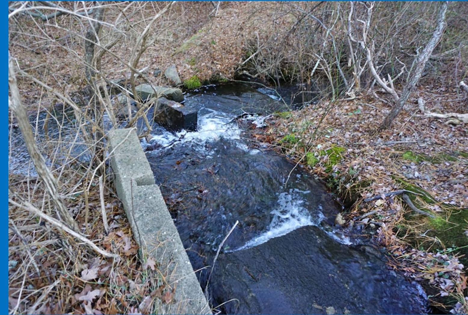
December 2018 – Old Spillway
