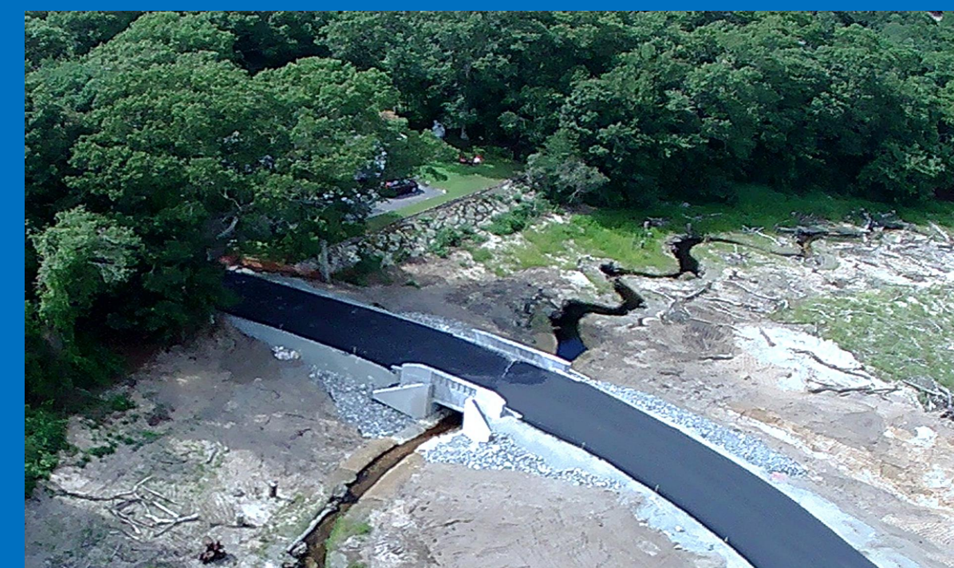
August 2021 – Road Paved
