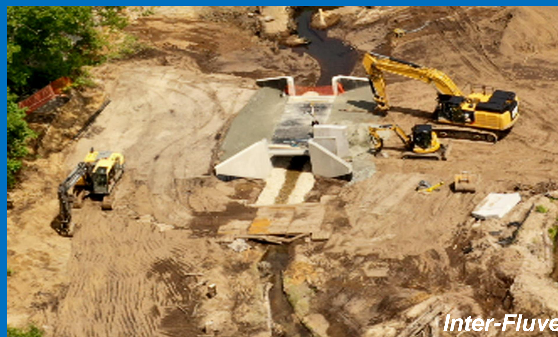
June 2021 – Construction of New Road
