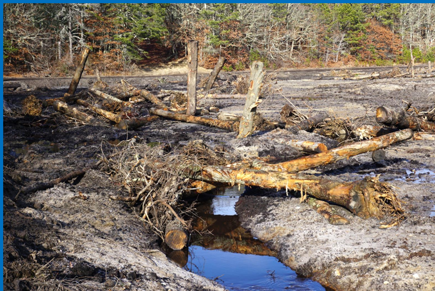
January 2021 – Logs & Root Wads Protect the River and Aquatic Life
