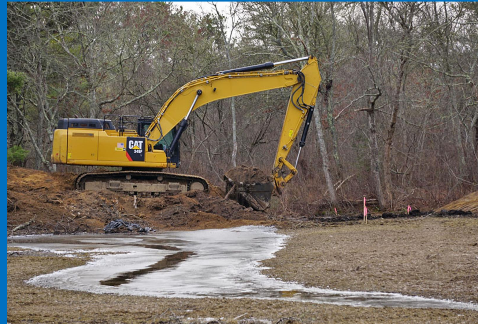
January 2021 – Dam Removal
